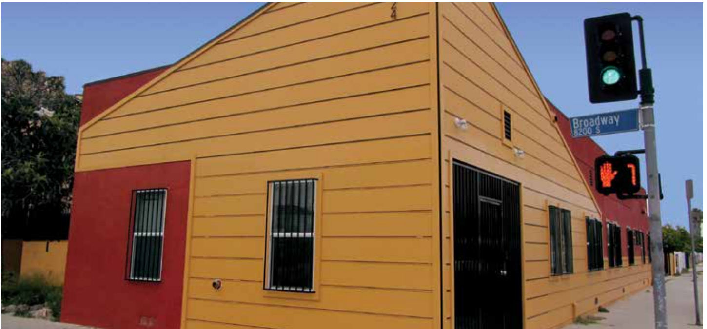
Main entrance, Family Emergency Shelter in South Los Angeles.
